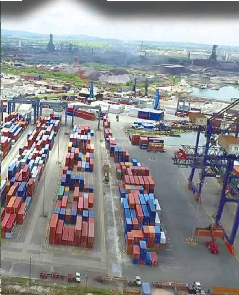
AFTER Port of Point Lisas Berth 5 Today
