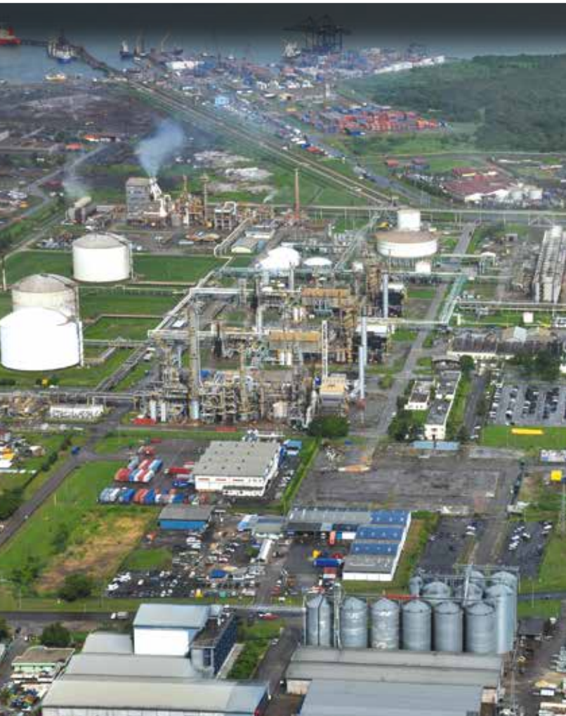
AFTER Industrial Estate Today
