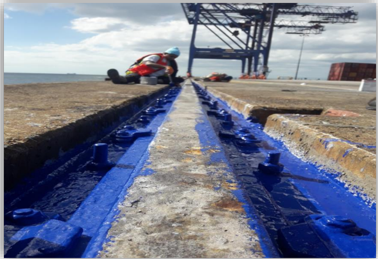
Corrosion repairs to Gantry Crane Rails
