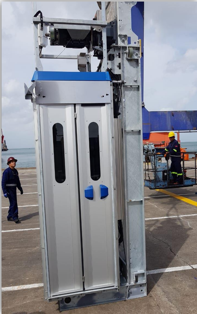
Replacement of defective elevator on Gantry Crane #1
