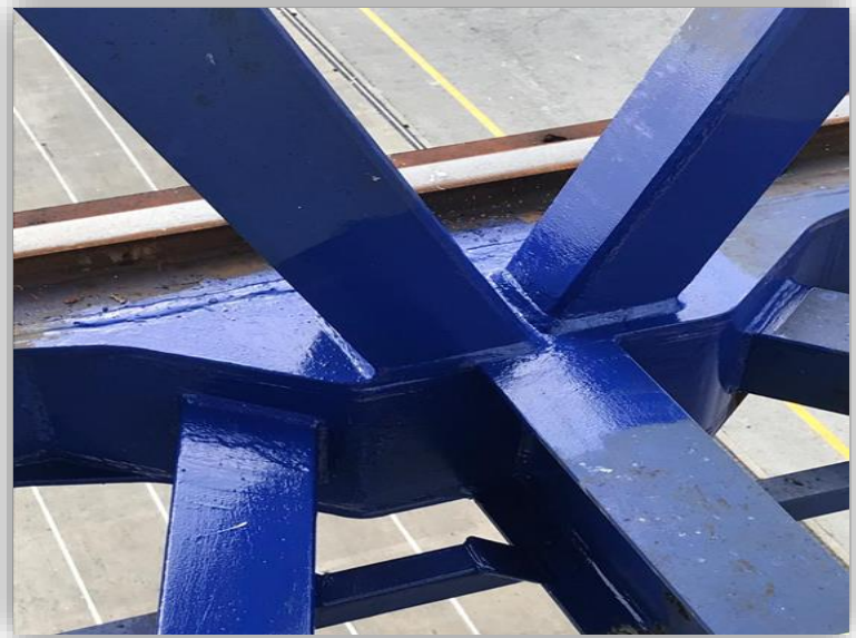
Corrosion repairs to Boom on Gantry Crane #1
